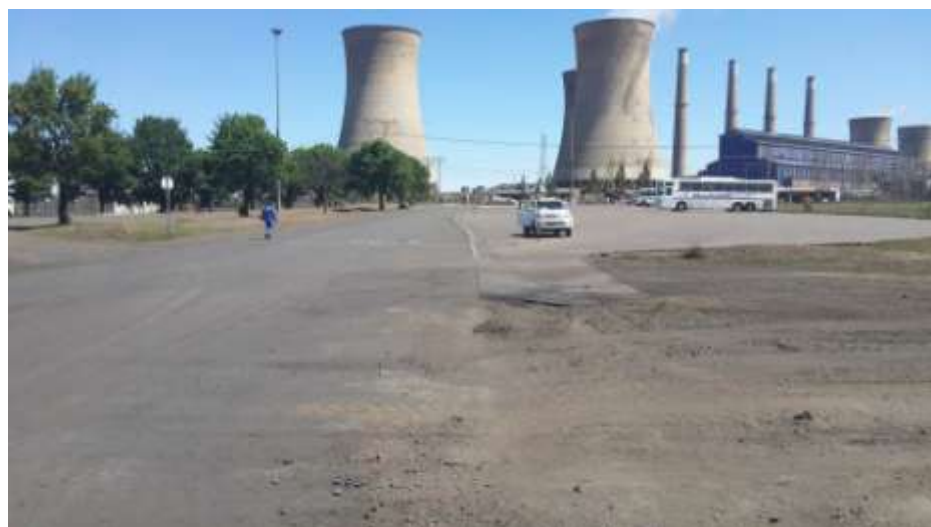
Four-way stop at intersection of Eike Avenue and the haul road
