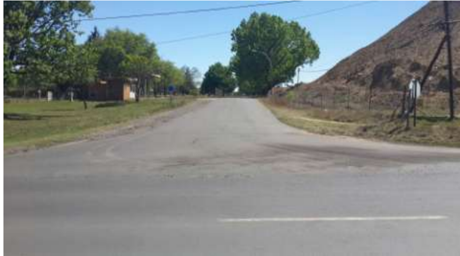
Camden Village access road from Eike Avenue
