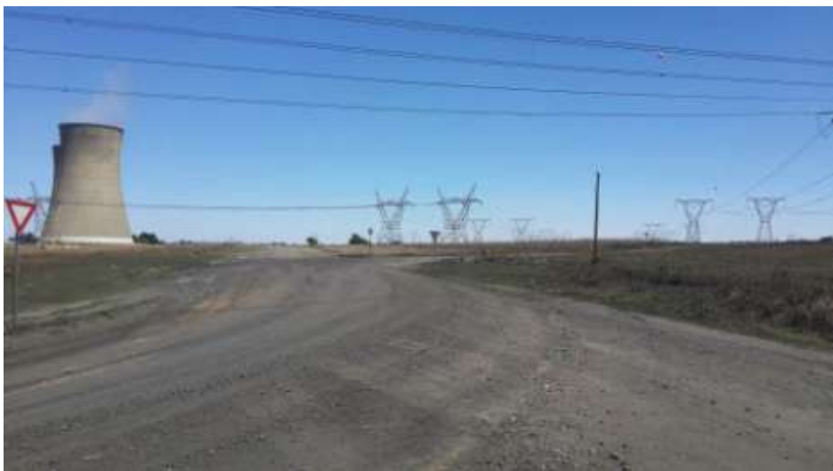
Intersection Road A and Road B near ash disposal facility camp site
