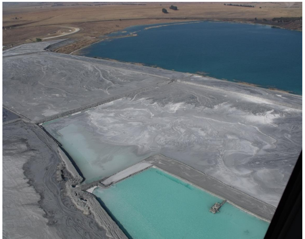
The existing ash disposal facility at the Camden power station.
