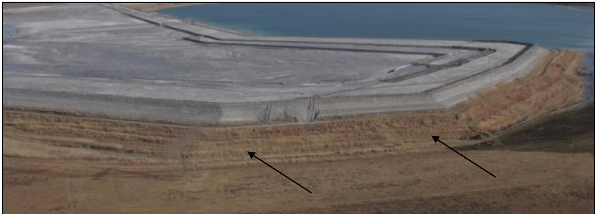
Figure 6-7: Capping on the existing ash disposal site in the foreground
