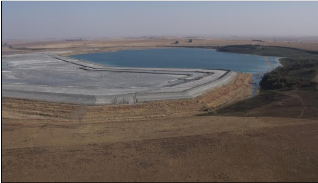
Figure 6-3: View of the sides of the existing ash disposal site
