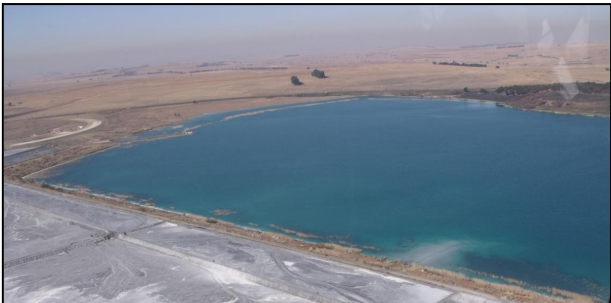
Figure 8-21: De Jager's Pan with the existing ash facility in the foreground
