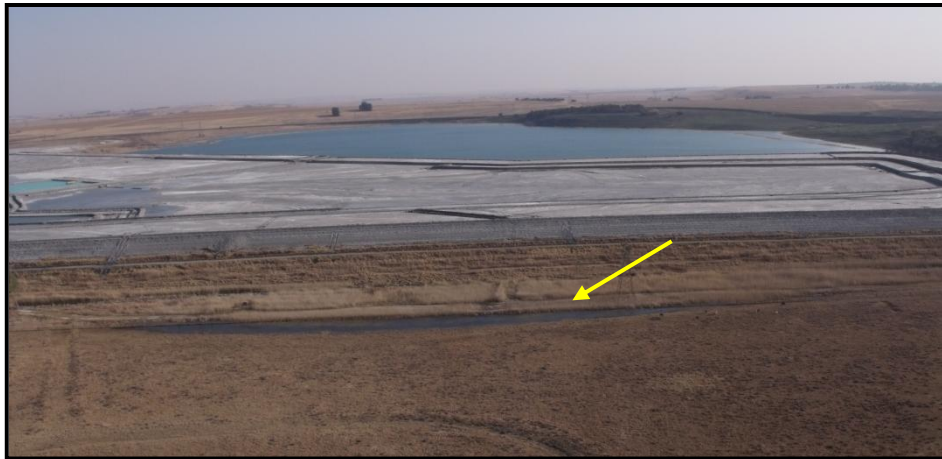
Figure 8-23 Drainage around the existing ash facility
