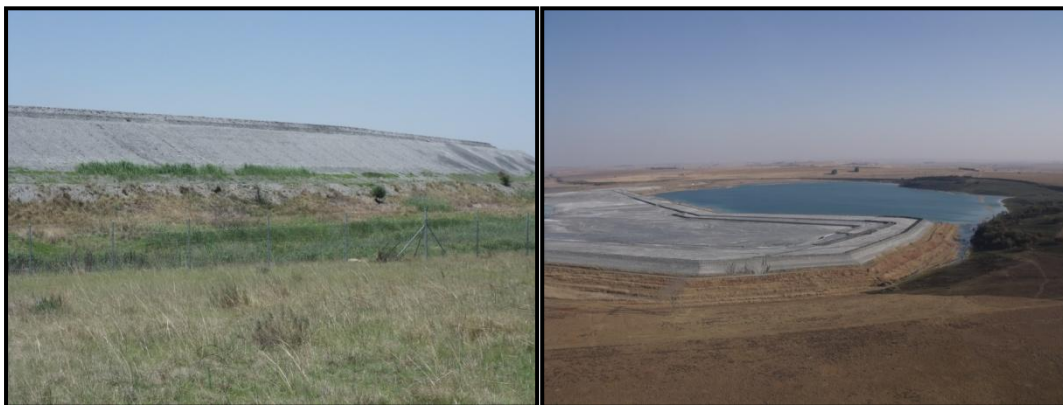
Figure 8-28: Difference in view from below (left) and above (right)
