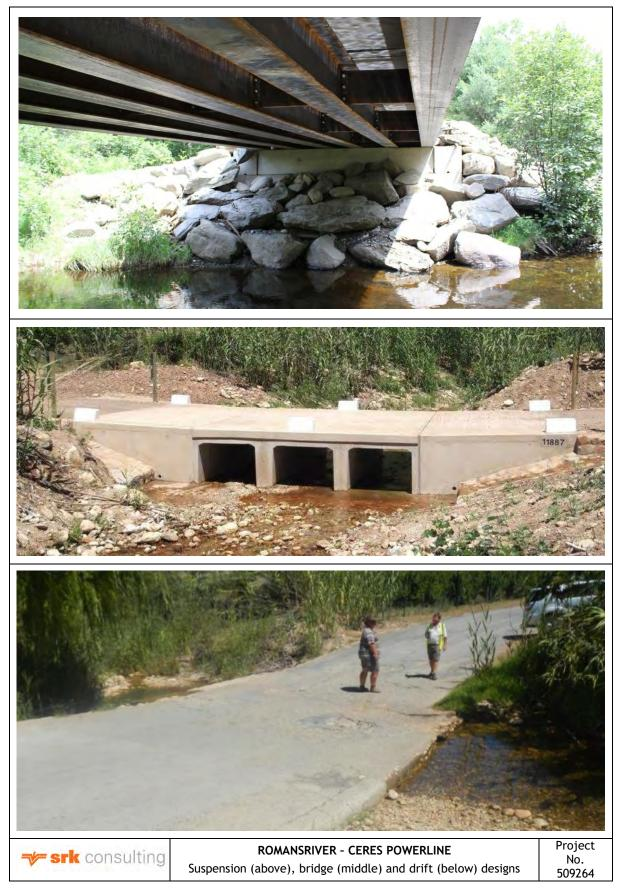
Figure 3-2: Suspension, low-level bridge and low level drift bridge designs
