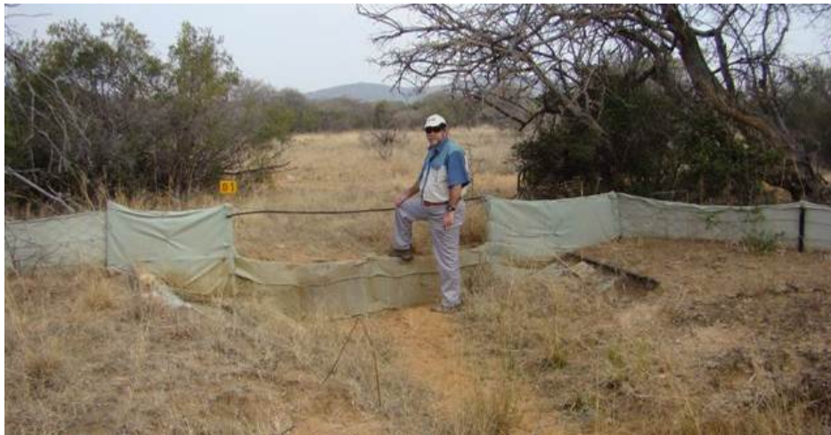
Figure 29: Silt screen application [32]
