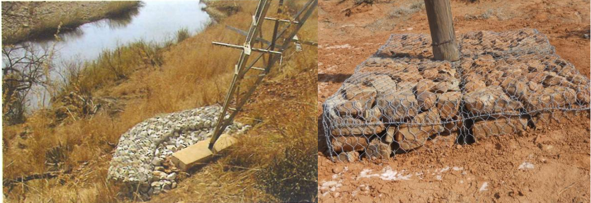
Figure 25: Gabion wall protecting tower leg and pole foundations [17], [28]
