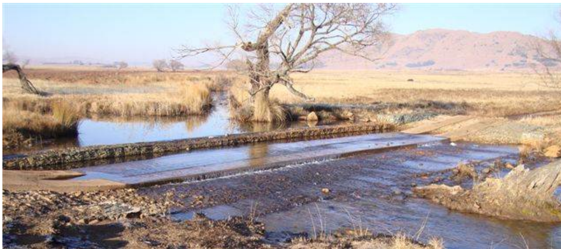
Figure 13: Reno Mattress drift crossing with concrete strips [32]
