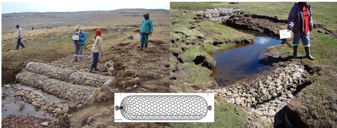
Figure 23: Sack Gabion weirs [32]
