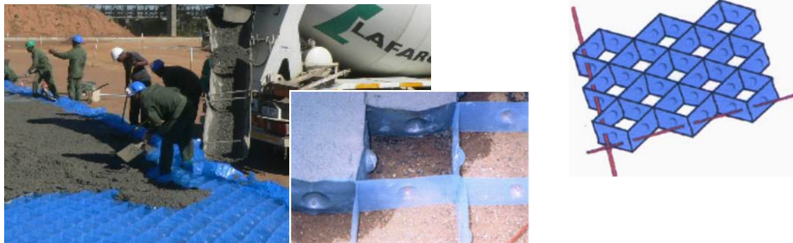
Figure 14: Geocells used with concrete (Hyson Cells 22 )
