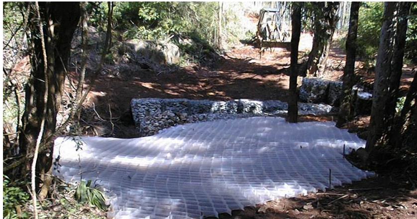
Figure 15: Geocells used as an approach to a low level pipe crossing [13]
