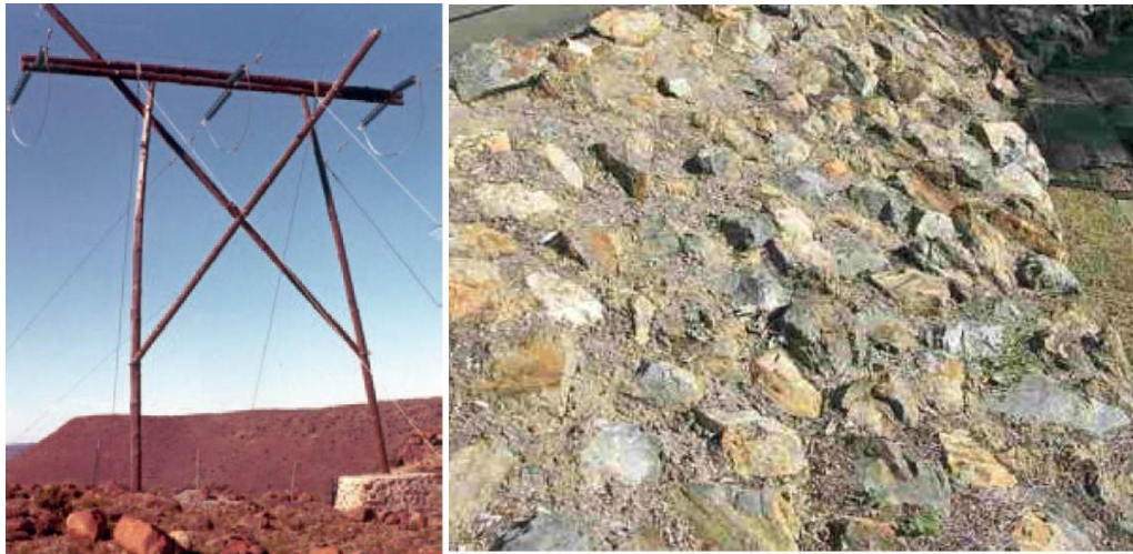
Figure 26: Stone pitching used as protection of wood pole [27, 26]
