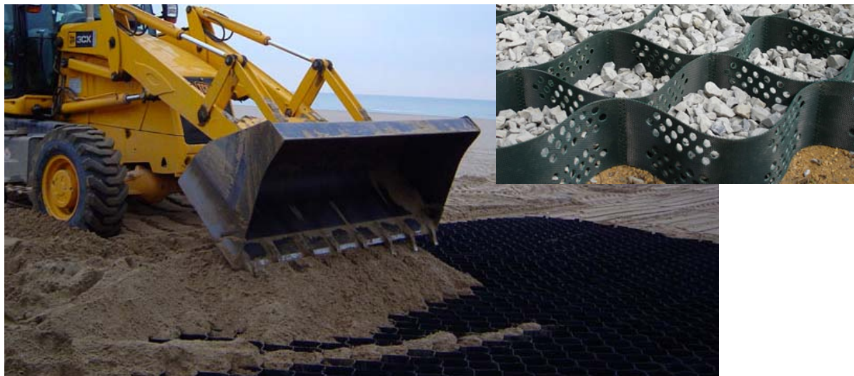
Figure 11: Temporary dry river bed or marsh crossing (30,31)
