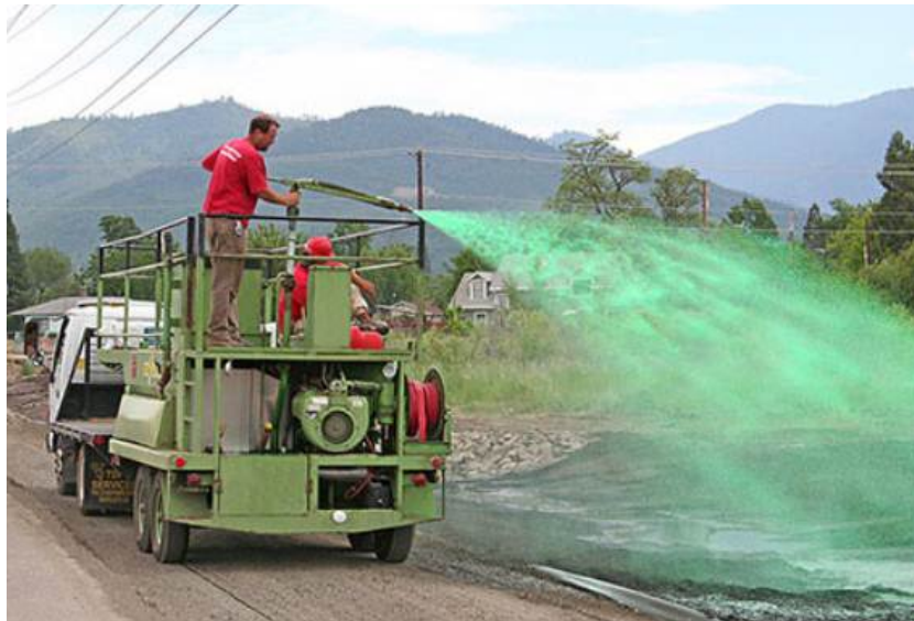
Figure 21: Application of hydroseeding [23]
