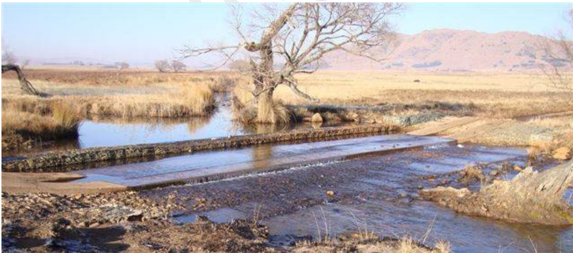
Figure 4-8: Reno mattress drift crossing (1)
