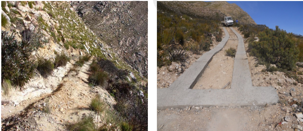
Figure 3-8: Concrete strip road before and after
