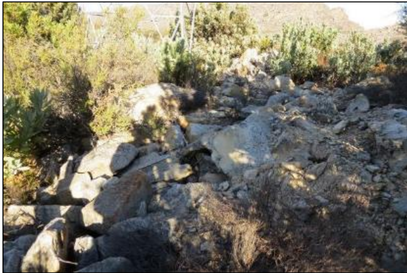
Figure 7. Piles of excavated rock smothering natural vegetation next to a pylon results in long-term loss of vegetation. Such events should be avoided by removing the material from the site.
