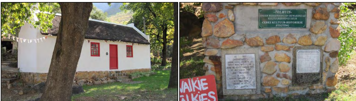
Plates 3.6 and 3.7: The old toll house and signage
