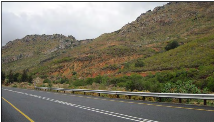
Plate: 4.14: A section of the route along the R43
