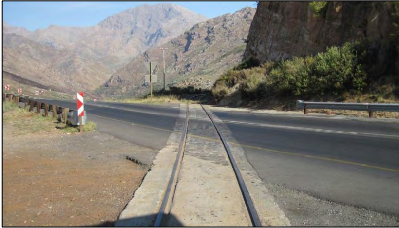
Plate: 4.19: The railway line looking south west, has to this point been above and to the west of the Pass after which it is below and east of the Pass before exiting the valley through a tunnel into Ceres
