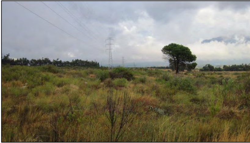
Plate: 4.13: Looking south along the existing Romansrivier to Tulbagh 132 kV powerline seen at left on metal Lattice towers.
