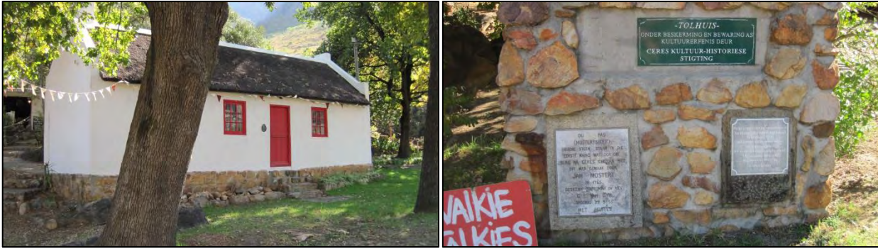
Plate 4.3: The Old Toll house. Plate 4.4: Various signs with very basic information acknowledging Mostert's old wagon road, Michell's Pass and the Toll House.
