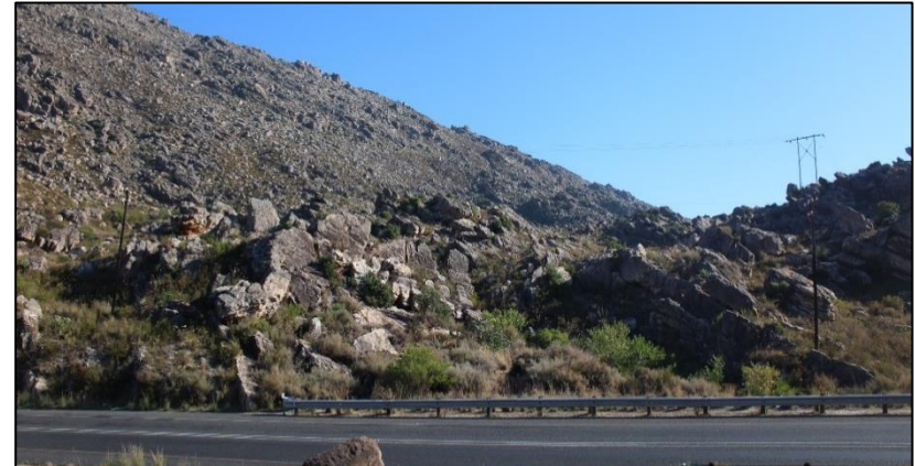
Figure 5-6: Proposed location of the powerline as it crosses the R46 between pylon 58 and pylon 59
