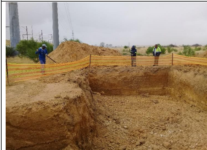
Figure 5: View of excavation being demarcated.
