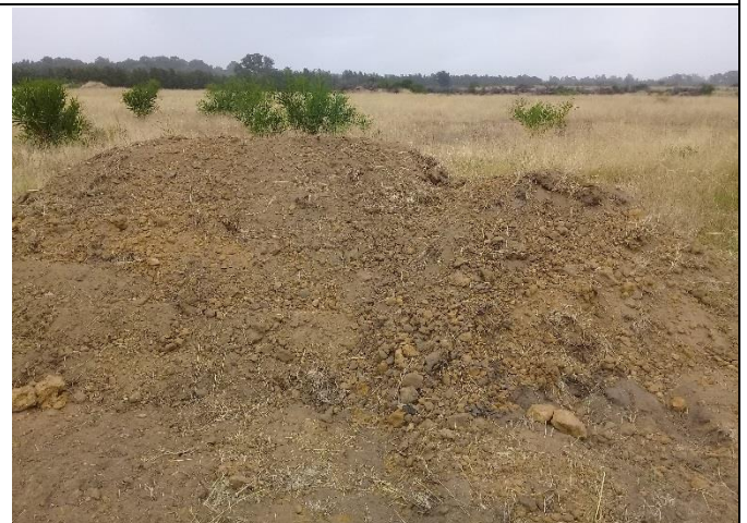
Figure 6: Topsoil stockpile separated from subsoil. Contractor must ensure that construction vehicles do not drive over it.
