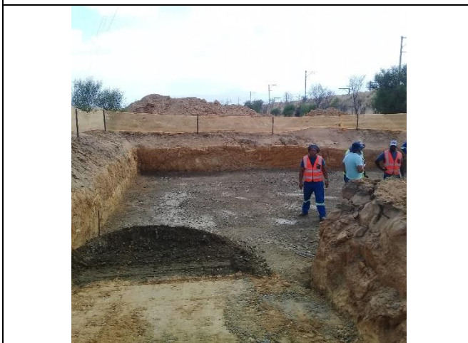
Figure 5: Monopole structure across the railway line being compacted.
