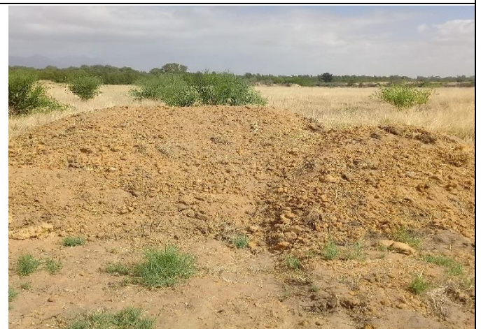
Figure 4: Topsoil stockpile separated from subsoil. Contractor must ensure that construction vehicles do not drive over it.
