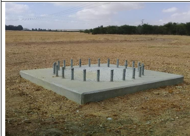
Figure 3: Completed and backfilled mono-pole structure.
