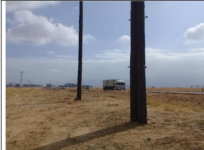
Figure 1: View of completed and backfilled wooden structures near the R44 road.
