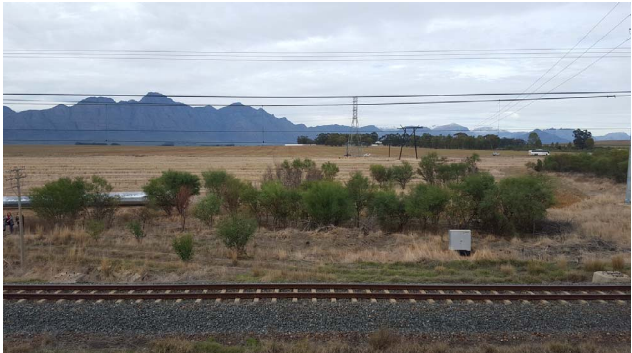
Looking over the site in a south-easterly direction. The route is to the left of the picture
