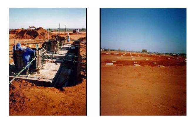
Photos 2 and 3: Example of transformer foundations
