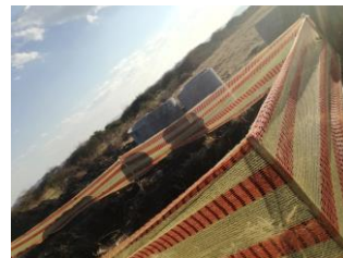
Photo8 Trenches and concrete slab for poles
