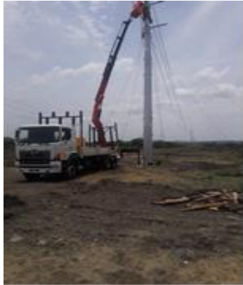
Construction activities on site: sagging and stringing
