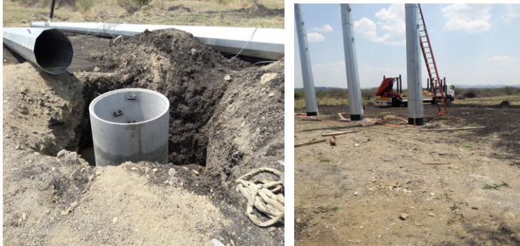
Construction activities at site
