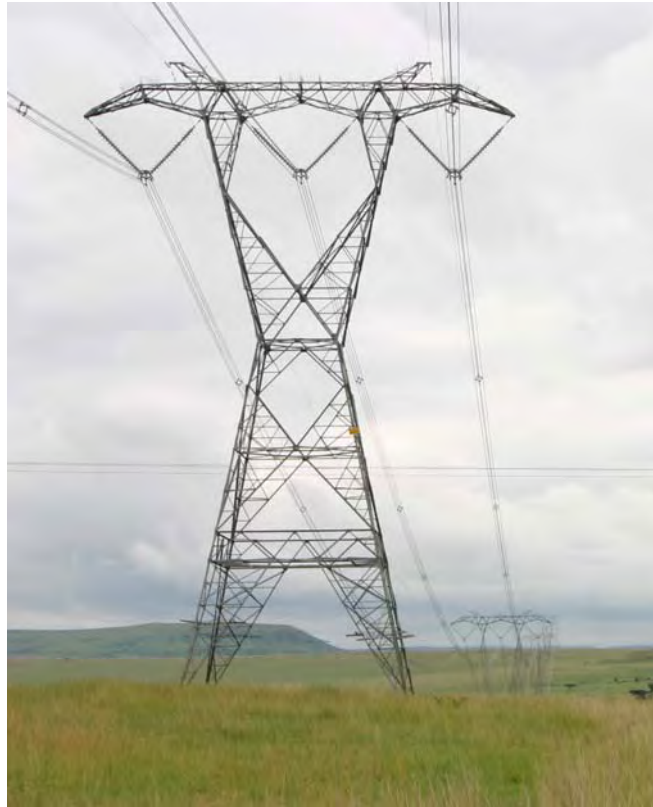
FIGURE 3.12 – 400KV TRANSMISSION POWER LINES - PHOTO OF STRAIN TOWER
