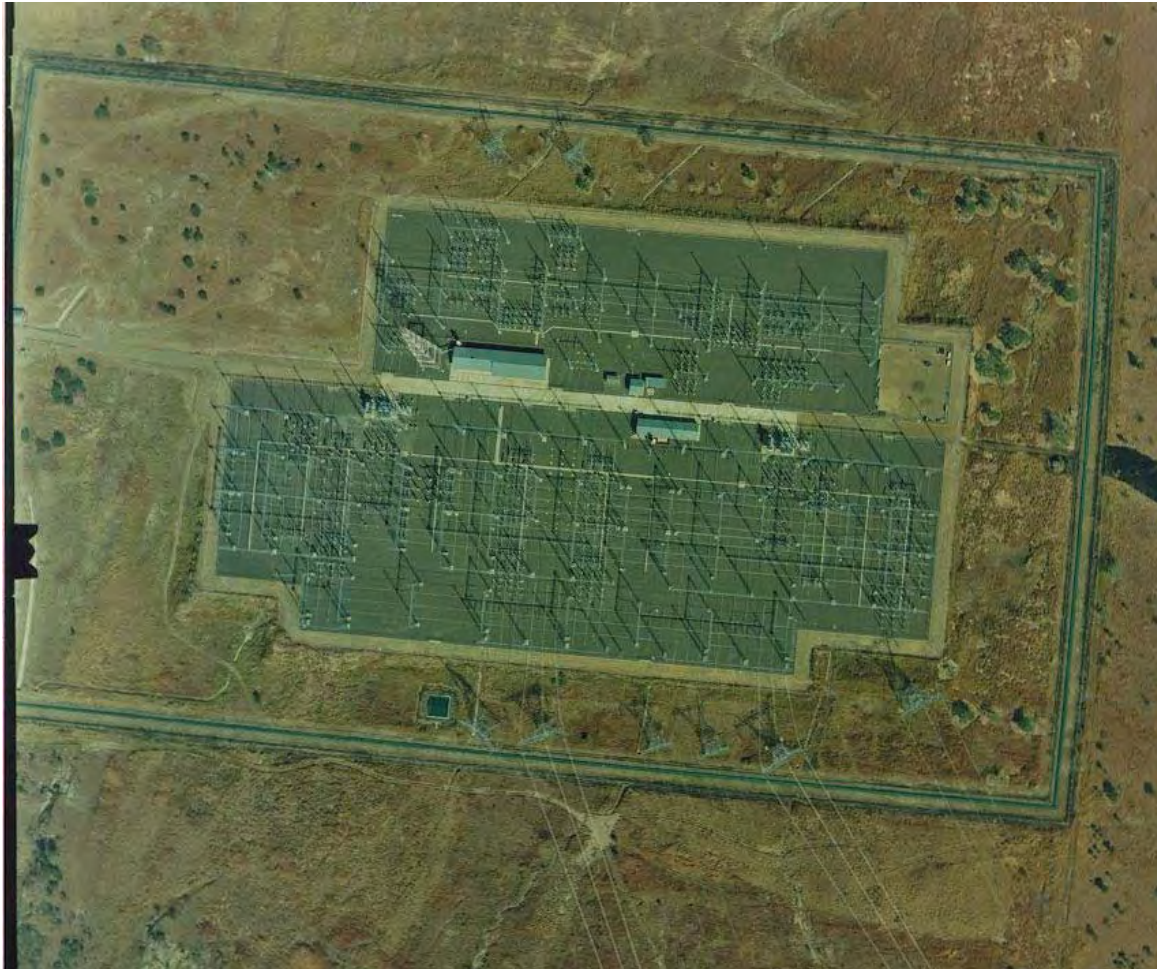
Figure 3.2 Example of Venus Substation (400kV), Estcourt, Kwa-Zulu Natal
