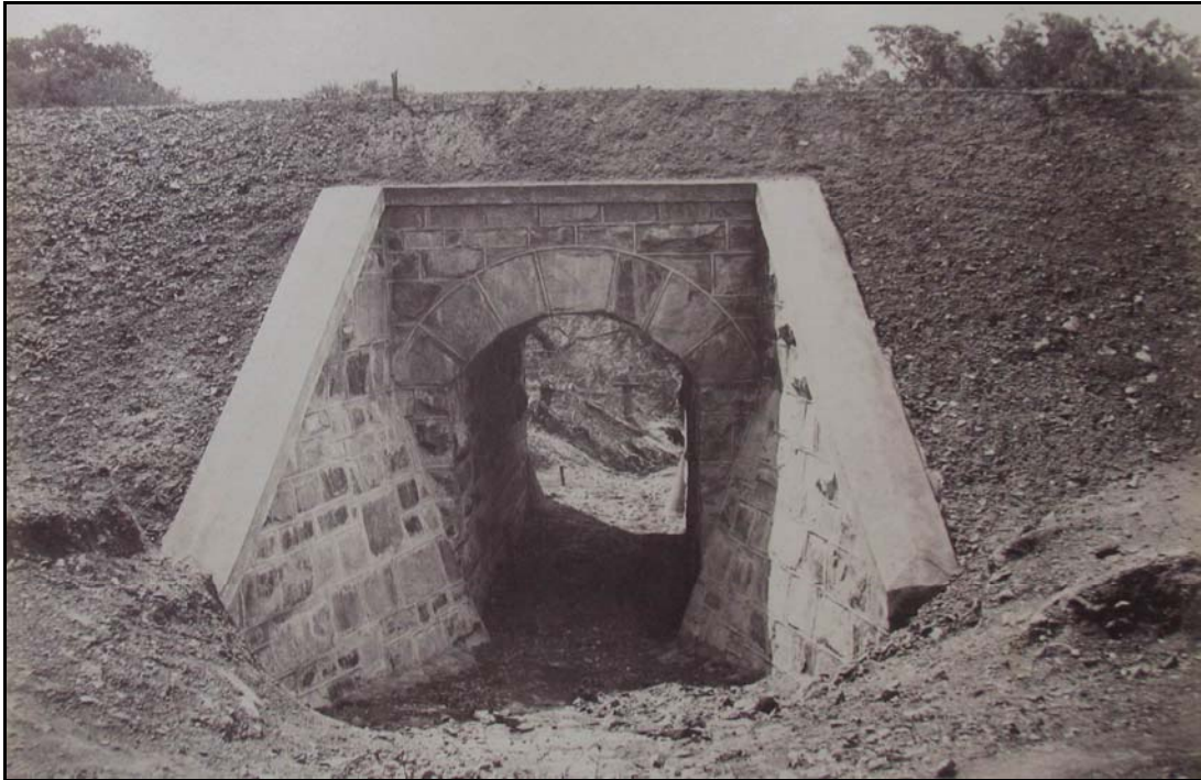
Plate 10: Photo of a culvert forming part of the Pretoria – Lorenço-Marques railway line shortly after completion
