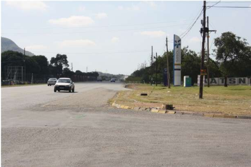
VIEW B: SOUTH EAST ALONG THE R511, TOWARDS WESTERN ROUTE AND DEVIATIONS
