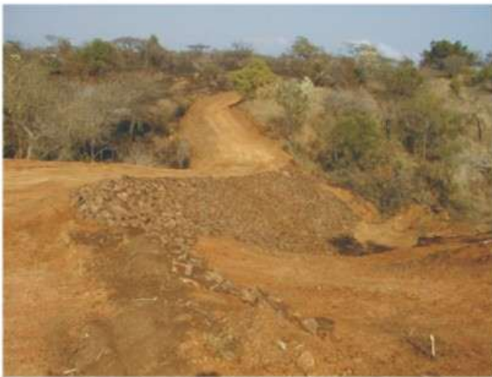
Example of bush clearing
