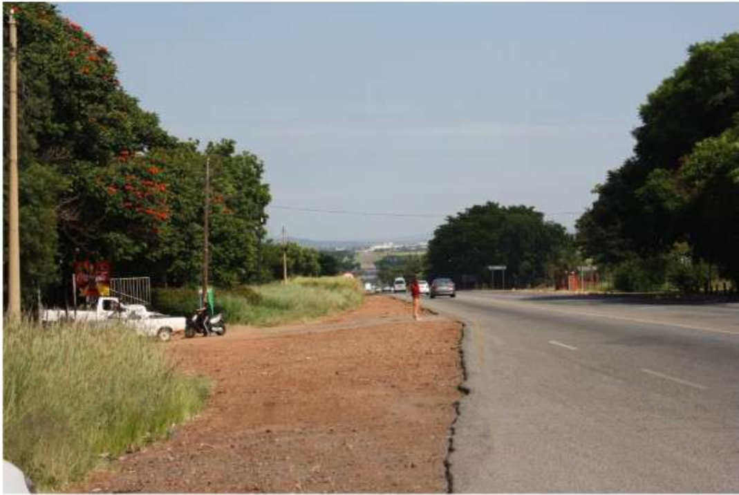
VIEW A: NORTH WEST ALONG THE R511, TOWARDS WESTERN ROUTE
