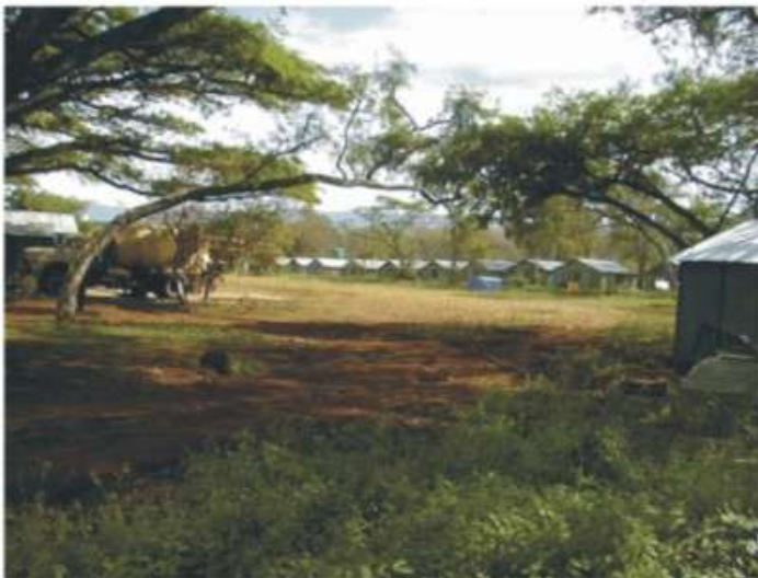
Example of a construction camp
