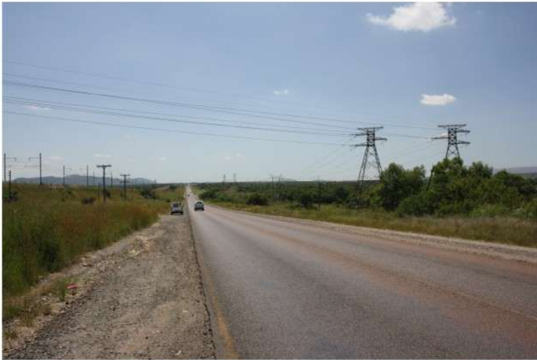
VIEW K: VIEW FROM R566 TOWARDS EASTERN ROUTE
