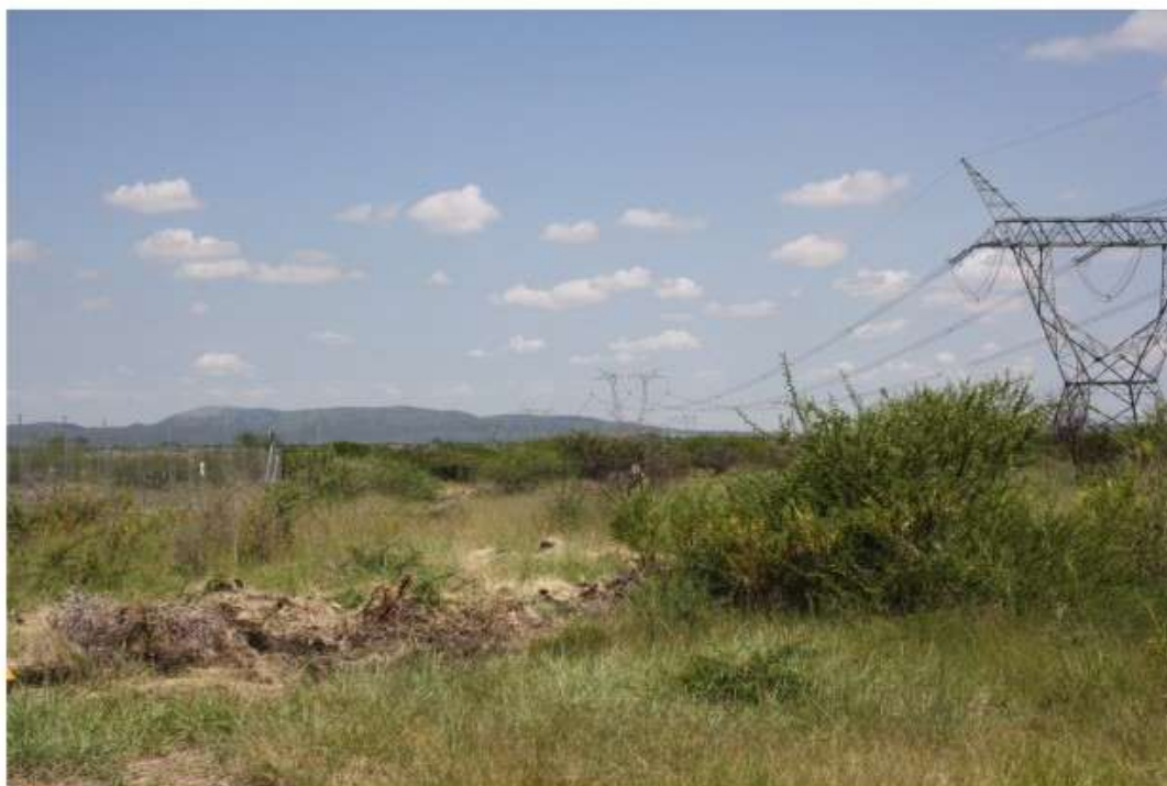
VIEW H: VIEW FROM DINALEDI SUBSTATION TOWARDS WESTERN ROUTE
