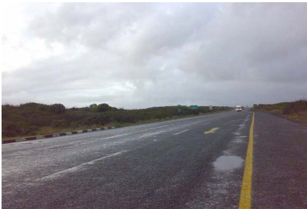
Photograph 5.1: R27 West Coast Road
