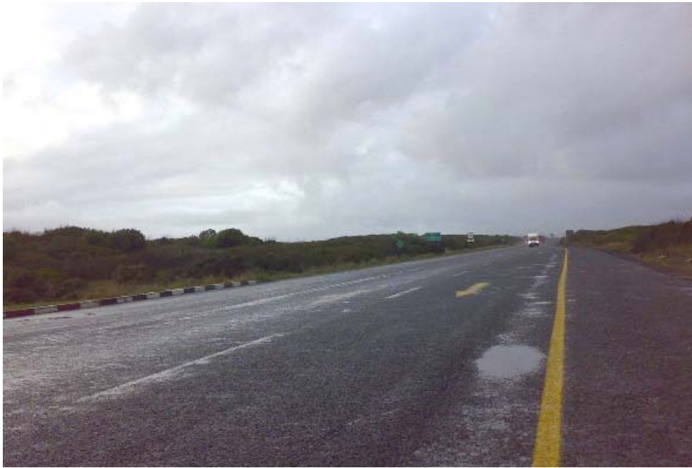
Photograph 5.1: R27 West Coast Road
