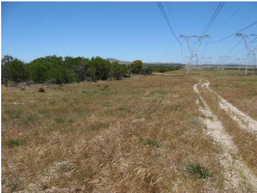
Plate 3: View of bushcut servitude on Koeberg – Stikland line (Alternative A; looking towards Omega site), with alien grasses dominant and Medium sensitivity vegetation remaining, with dense invasive Acacia saligna outside the servitude.
