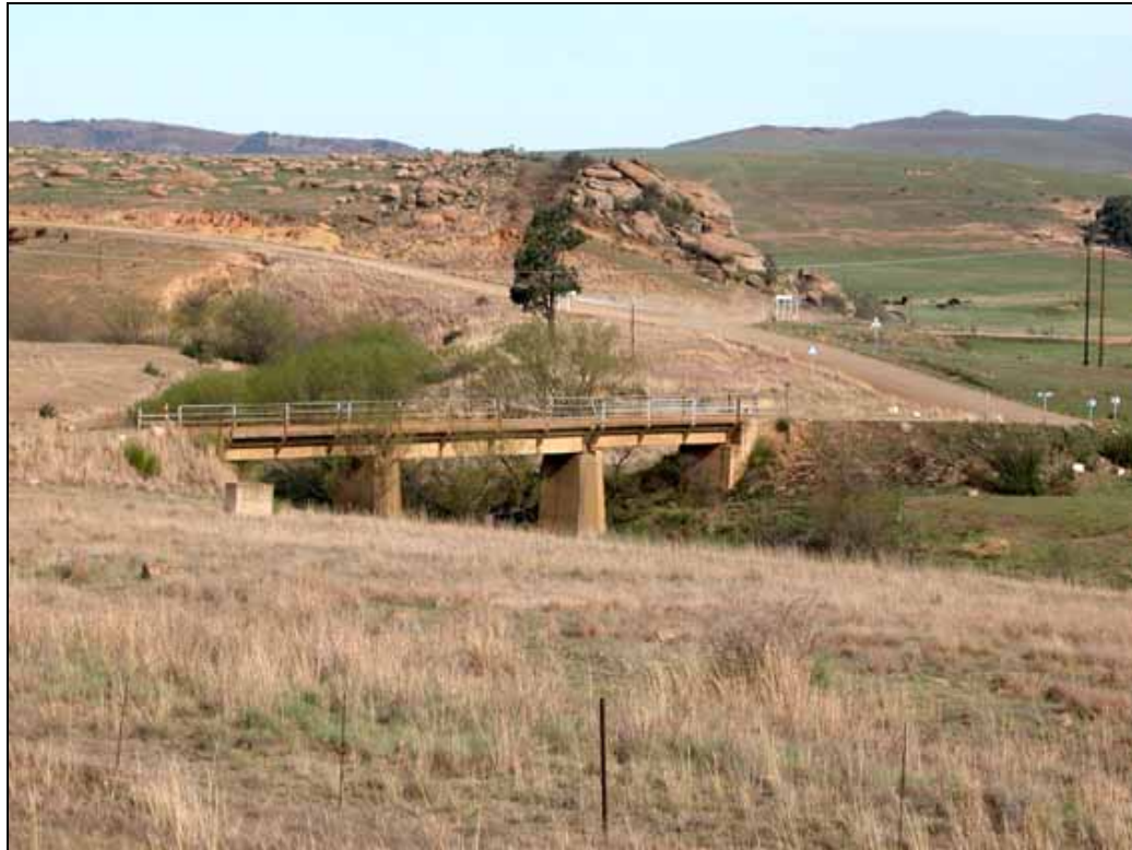
Plate 25 Present-day view of the bridge at Site BH18 .
