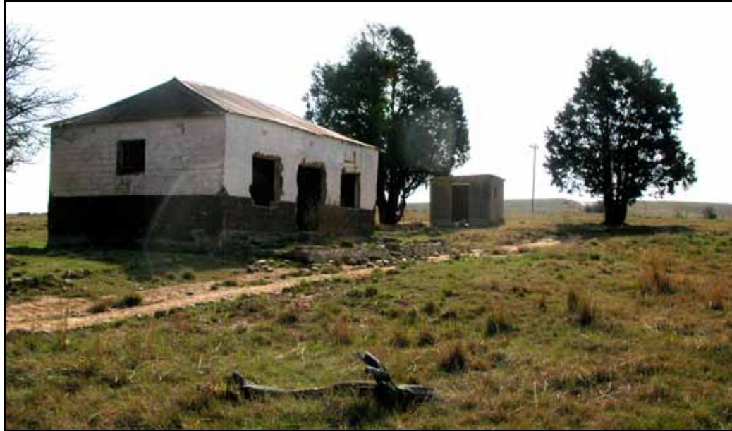
Plate 21 The building from BH14 .
