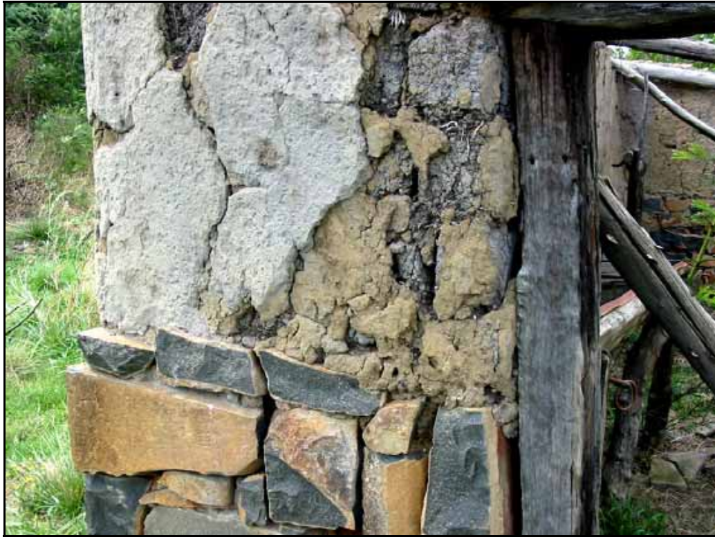
Plate 9 Close-up view of the stone structure with the mud brick extension ( deige ) on top.
