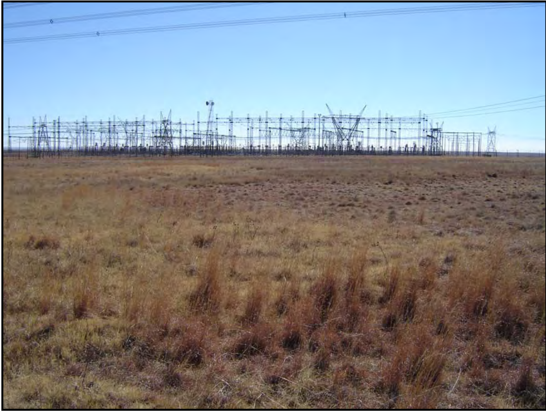
Photo 1: General view looking north over surveyed area
