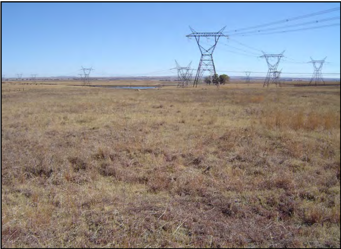
Photo 2: General view looking west over surveyed area
