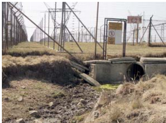
Figure 1. Outfall from substation.
