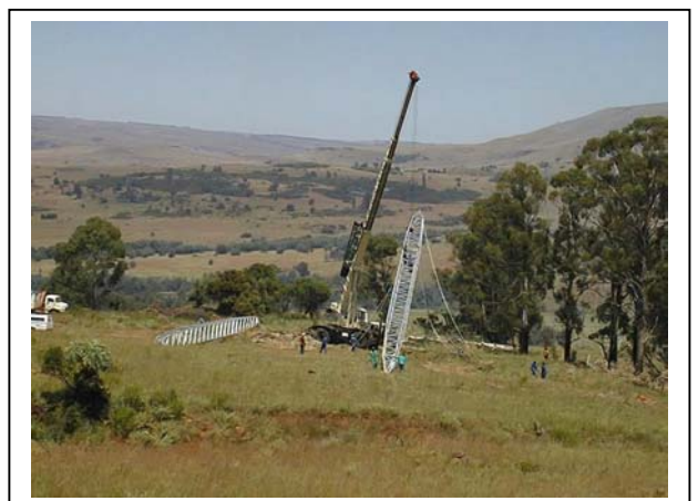
Photograph B6: Erection of towers by crane
