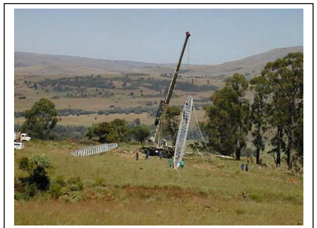
Photograph B6: Erection of towers by
