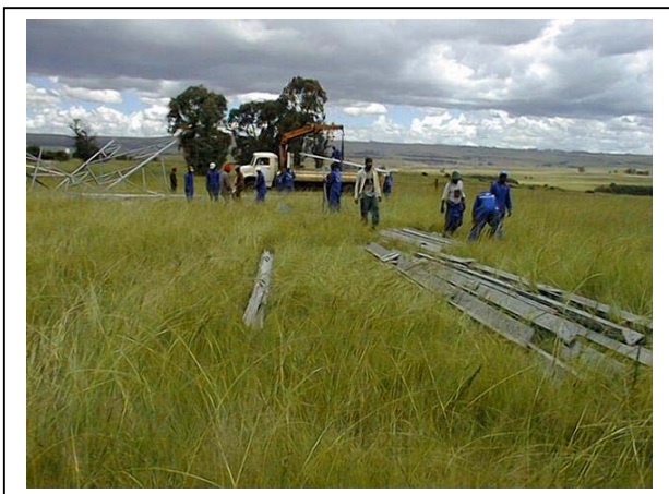
Photograph B5: Towers are erected on site
