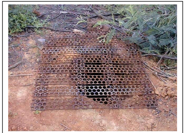
Photograph B4: Cover over foundations
