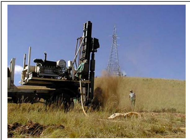
Photograph B3: Drilling of foundations
