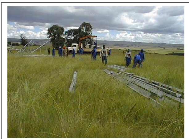
Photograph B5: Towers are erected on site
