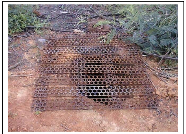
Photograph B4: Cover over foundations
