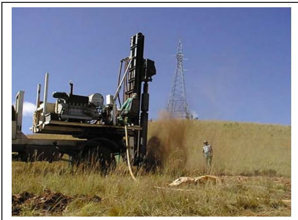
Photograph B3: Drilling of foundations
