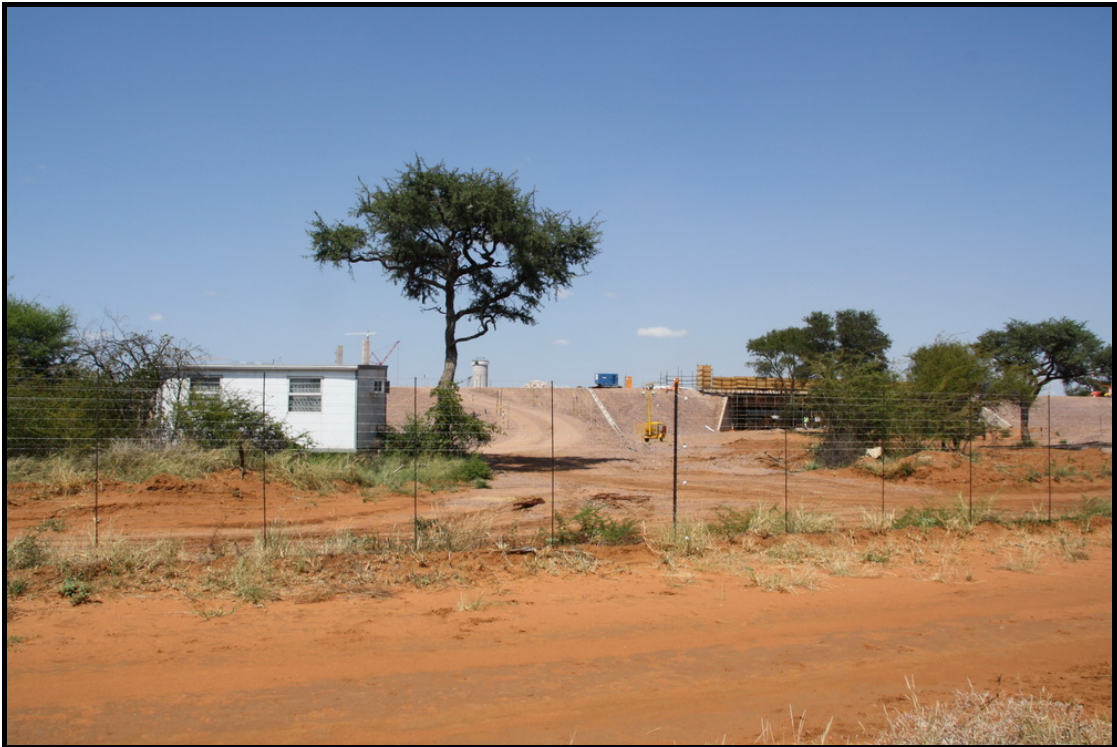
Fig. 4. Where the conveyor will cross into Medupi Power Station.
