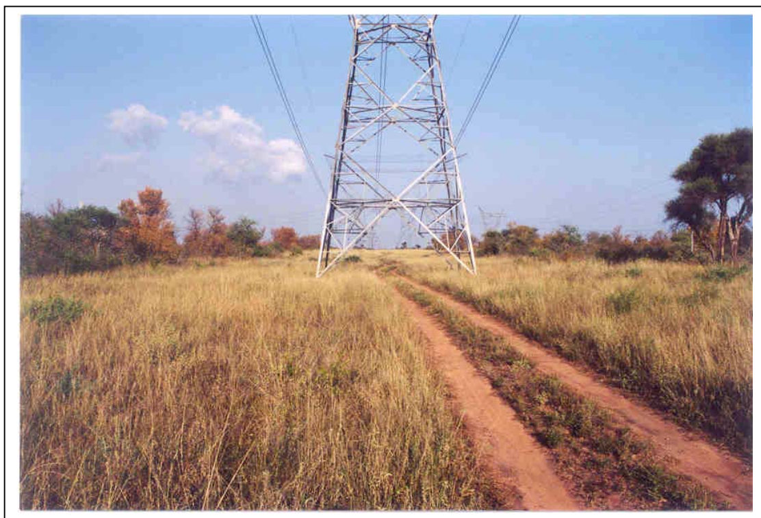
Photograph 20: Impact: placement of tower foundations
