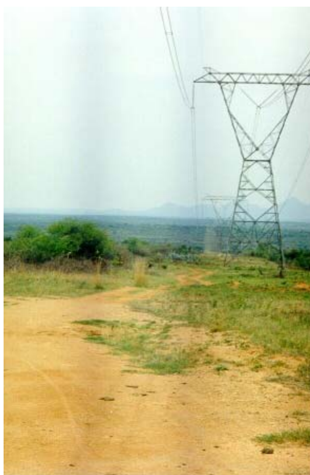
Plate 3 Existing 400 kV Transmission line near Pudiyakgopa. Uninterrupted vista with low vegetation promotes visibility of the towers
