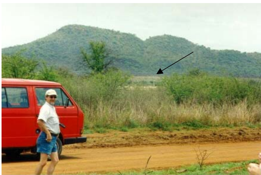
Plate 5 Mottled backdrop created by the relief and vegetation camouflages towers some distance away from the viewer. The arrow indicates approximate position of a tower of the existing Matimba-Witkop No 1 400 kV Transmission line
