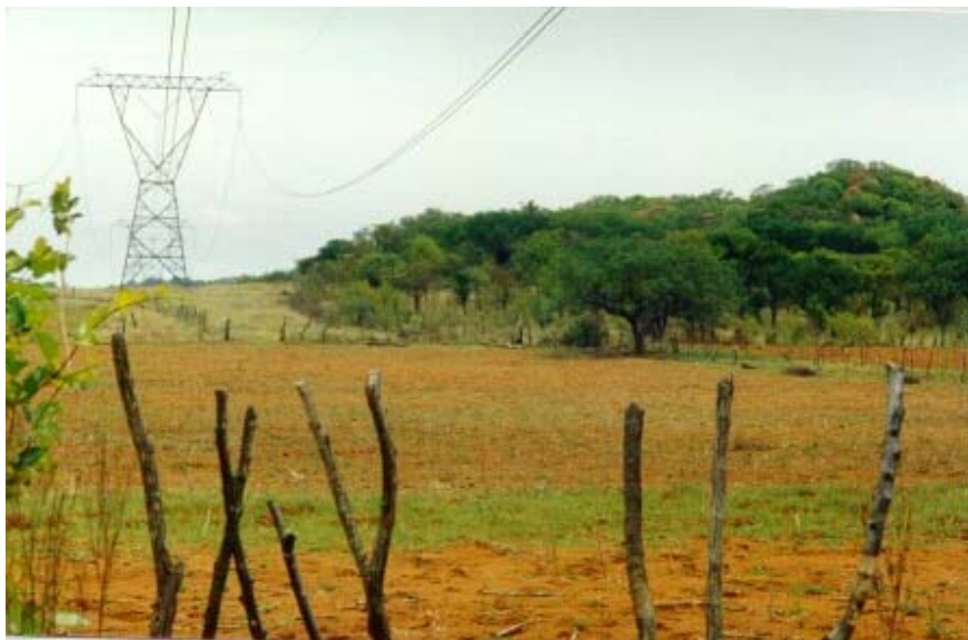
Plate 4 Change in vegetation and relief, from low bushes and flat topography to trees and higher relief reduces the potential for visual impact from a distance (existing 400 kV Transmission line tower)
