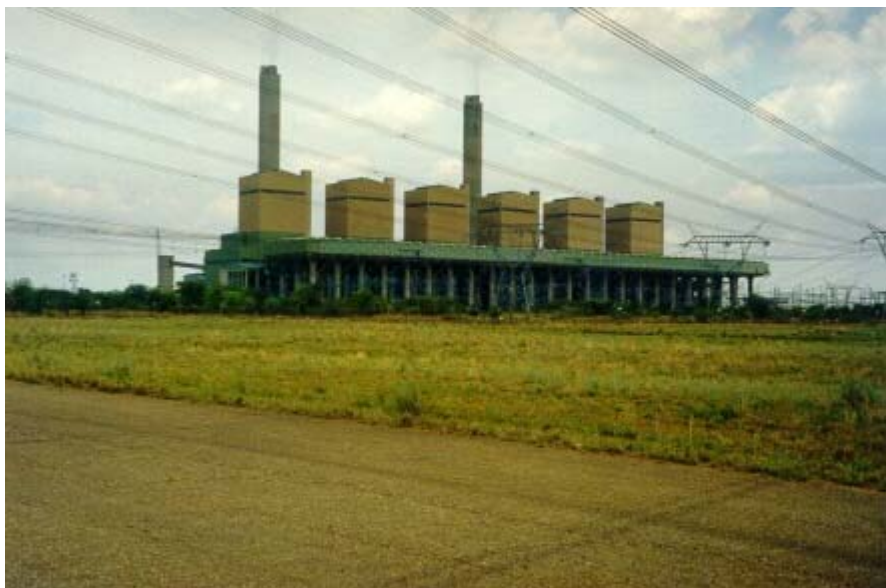
Plate 7 Matimba Powerstation , near Ellisras, with numerous overhead powerlines feeding out of the Matimba Substation
