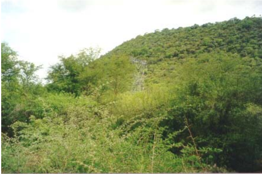
Plate 1 Tower of the existing 400 kV Transmission line against a mottled, vegetation backdrop near Moepel Farms
