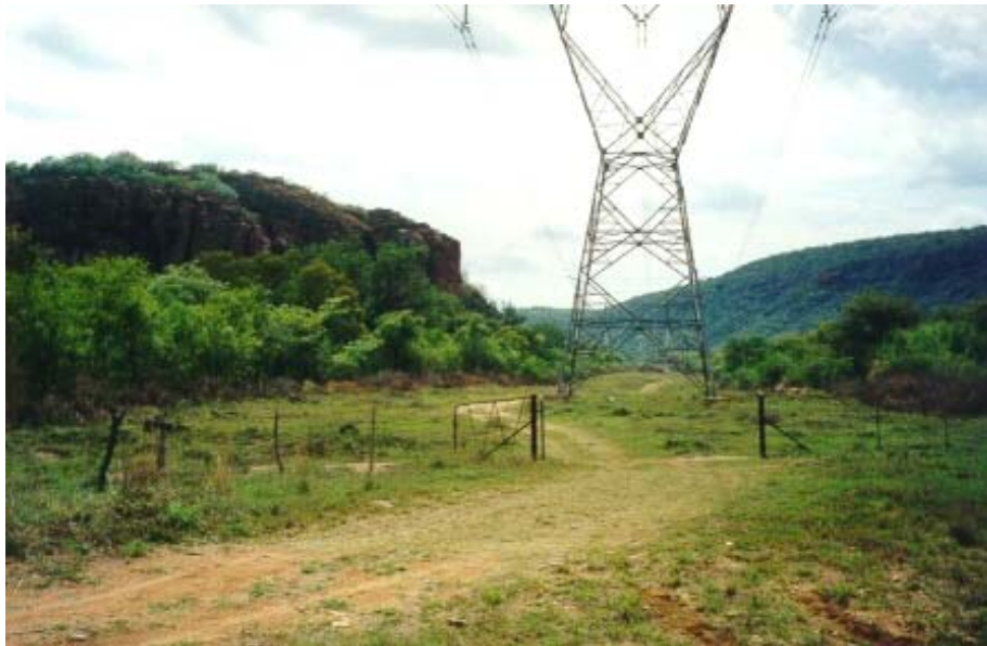
Plate 6 Existing 400 kV Transmission line passes through the nek between Moepel Farms and Masebe Nature Reserve
