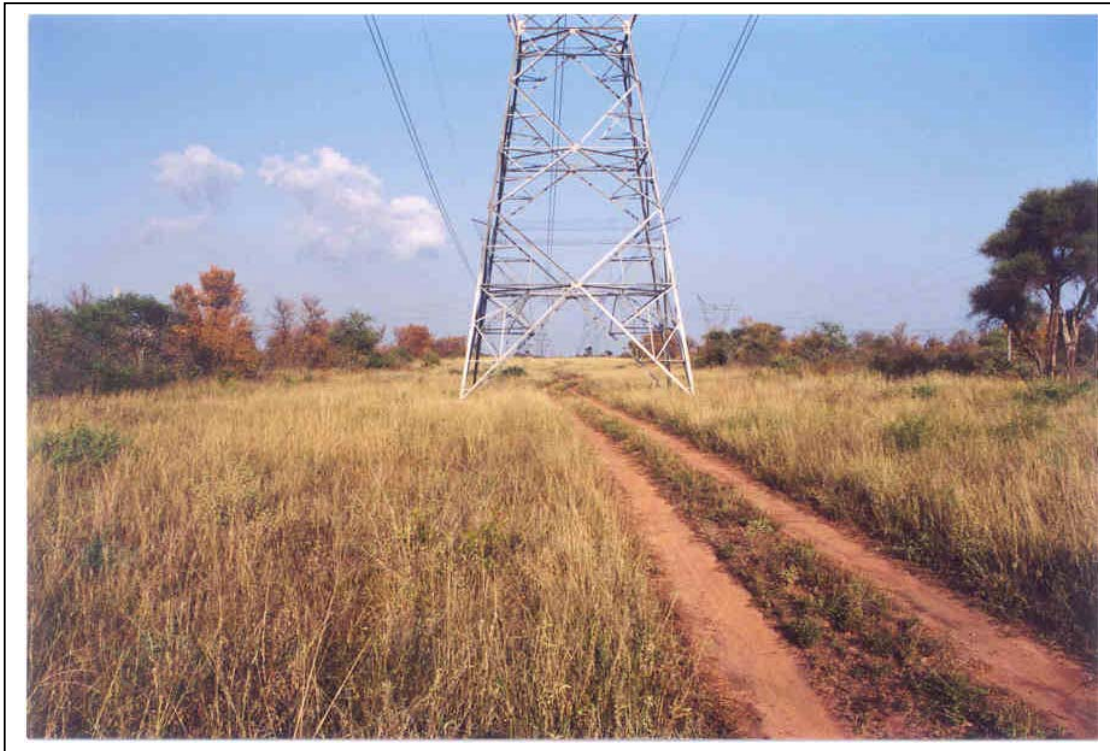
Photograph 20: Impact: placement of tower foundations
