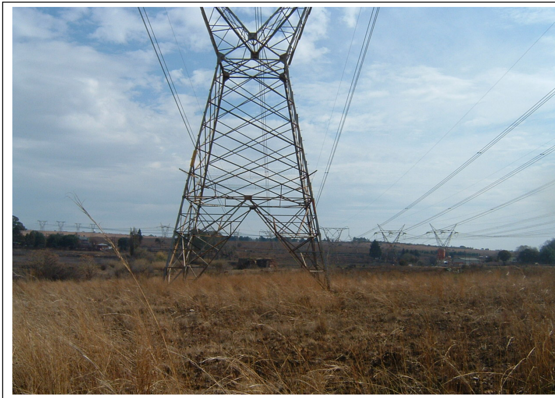
Figure 2- The existing 400kV Apollo-Pluto power from where a loop-in and loop-out power line will be established to the Verwoerdburg Substation (above).
