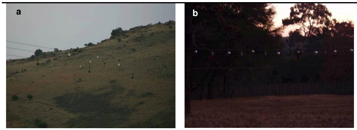
Figure 14: An example of the Inotec BFD88 diverter used alongside conventional dynamic devices (photographs courtesy of Chris van Rooyen).
