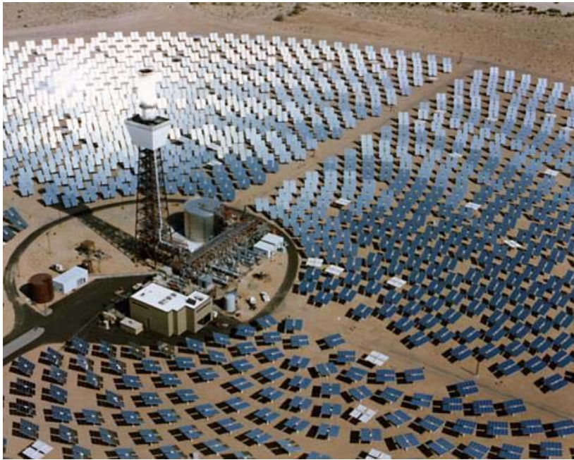
Figure 2: An example of a power plant using central receiver technology. This is a 10MW demonstration plant that was built in the United States – image courtesy NREL.
