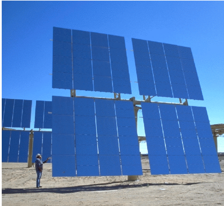
Figure 3: Single heliostat at roughly 130 \text{ m}^2 – image courtesy NREL
