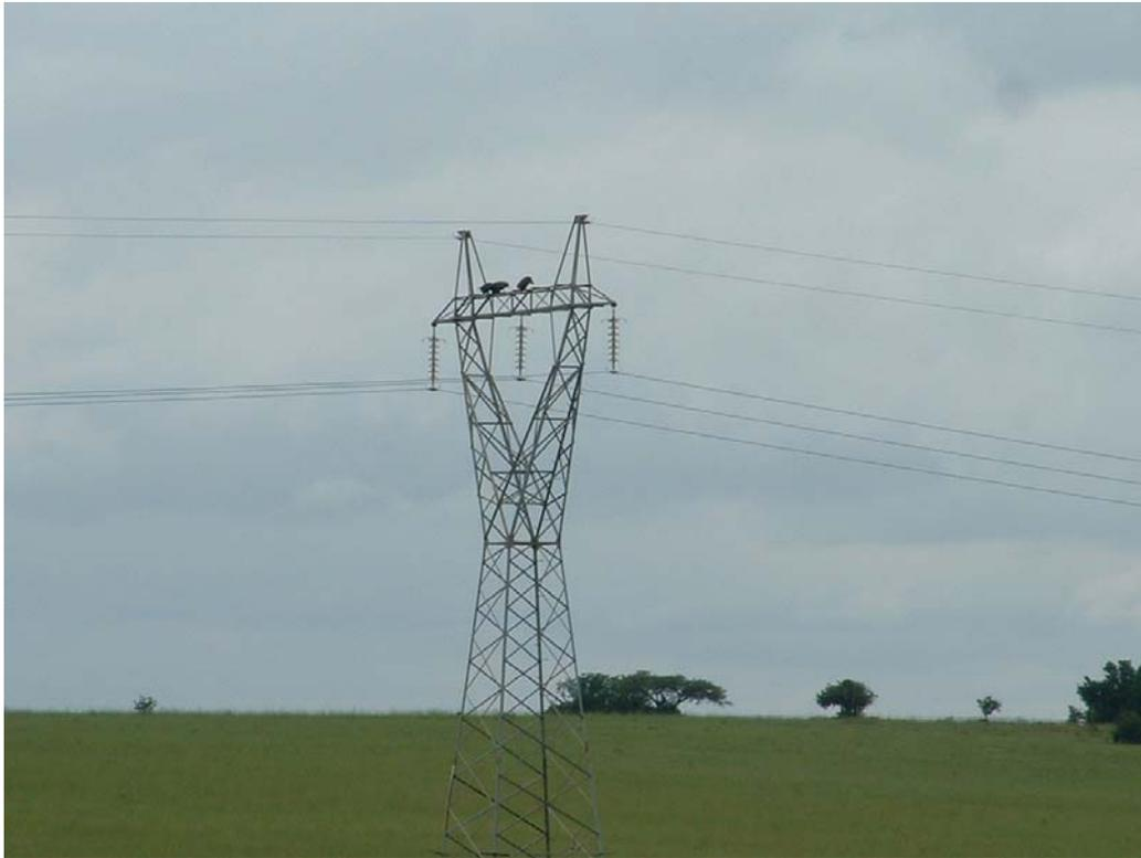
Figure 12: Photo showing Hadeda Ibises perched on a self-supporting 275kV power line tower, having the potential to cause bird streamer faults on the central phase.
