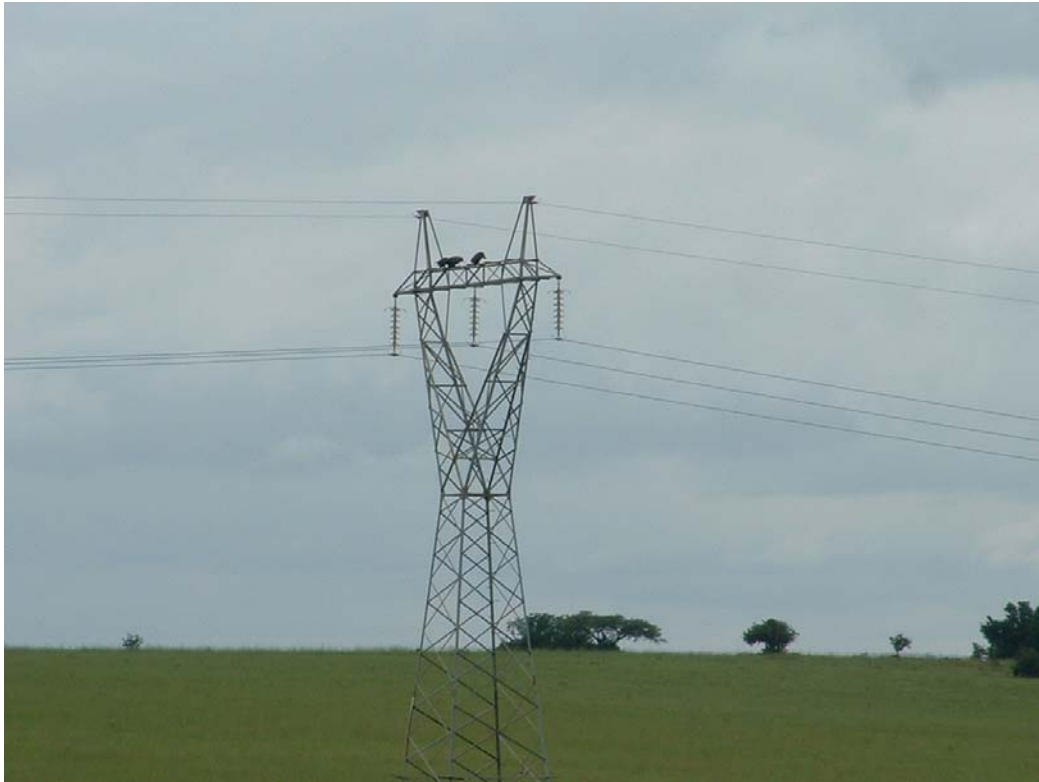
Figure 12: Photo showing Hadedda Ibises perched on a self-supporting 275kV power line tower, having the potential to cause bird streamer faults on the central phase.
