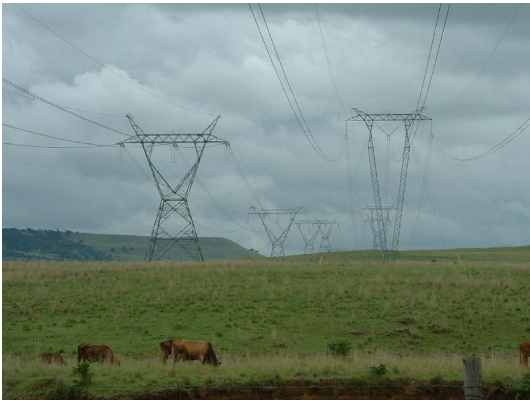
Figure 10: Photo showing the location of similar size power lines parallel to each other, thereby reducing the collision potential by keeping the disturbance in a single corridor.
