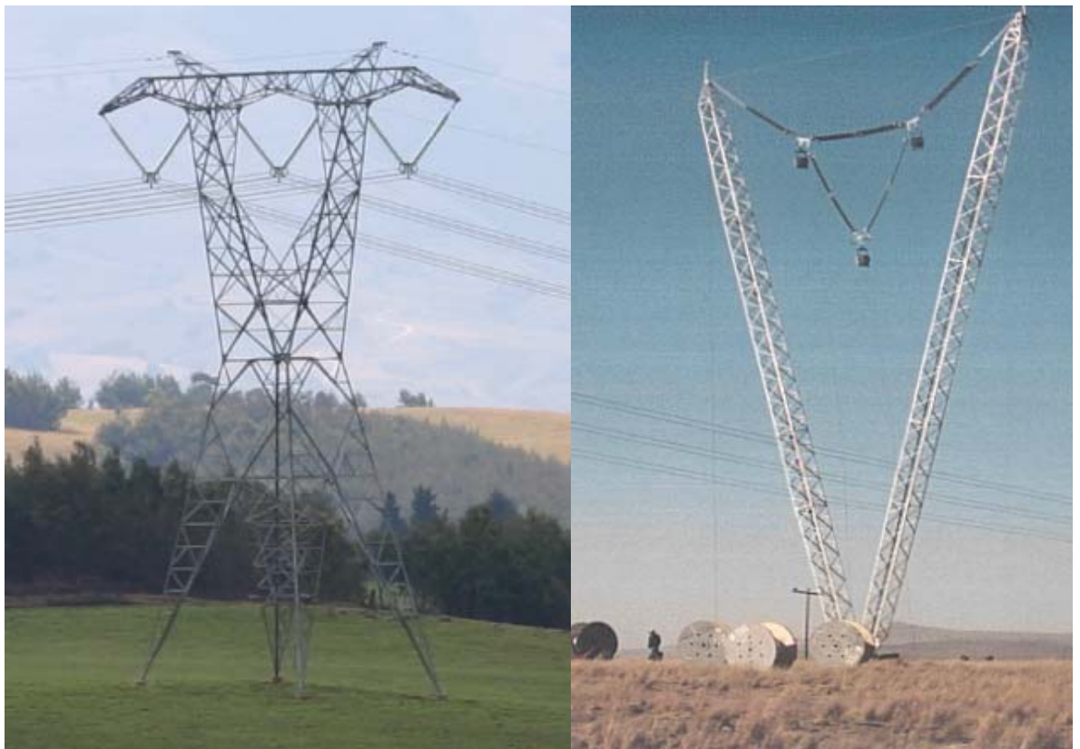
Figure 2c: Examples of both strain tower and compact cross rope suspension tower types
