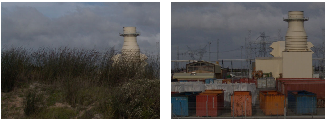
Photograph 9.2: Close views of the OCGT plant in Atlantis
