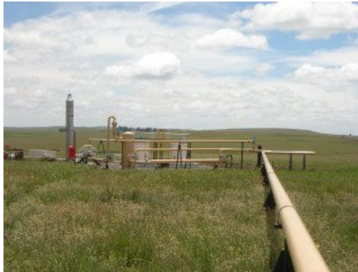
Photograph 9.1: UCG pilot plant on the farm Roodekopjes
