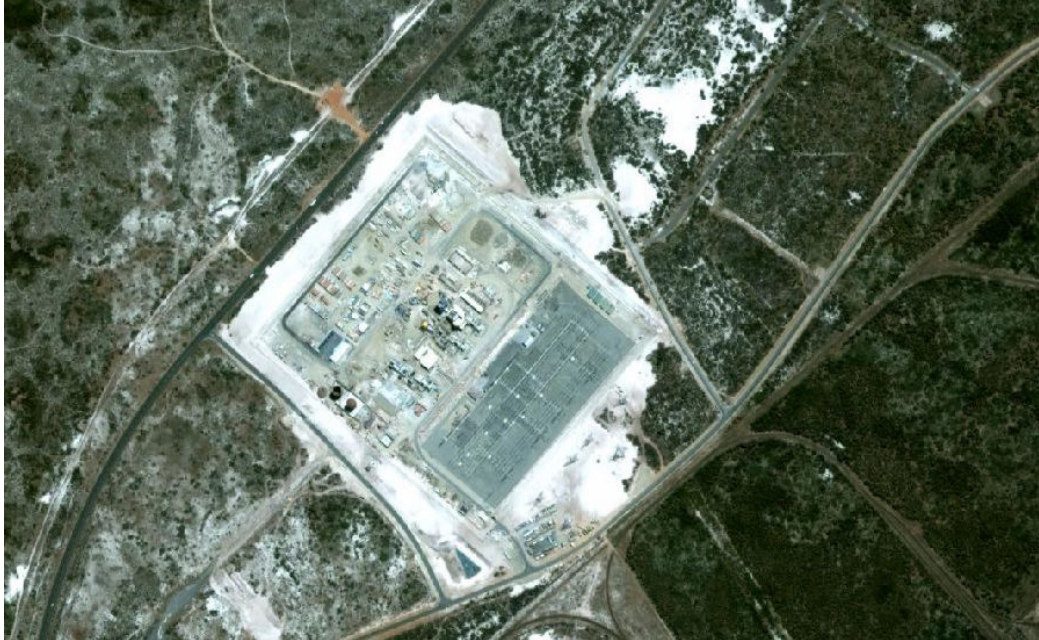
Figure 9.3: Aerial view of Atlantis OCGT (footprint 56 ha)
