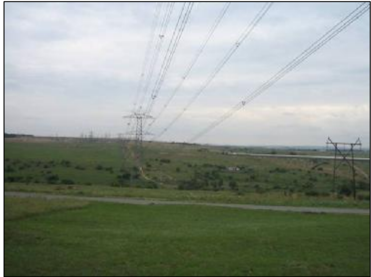
Figure 13: Land use surrounding the Lulumisa substation in the Diepsloot area
