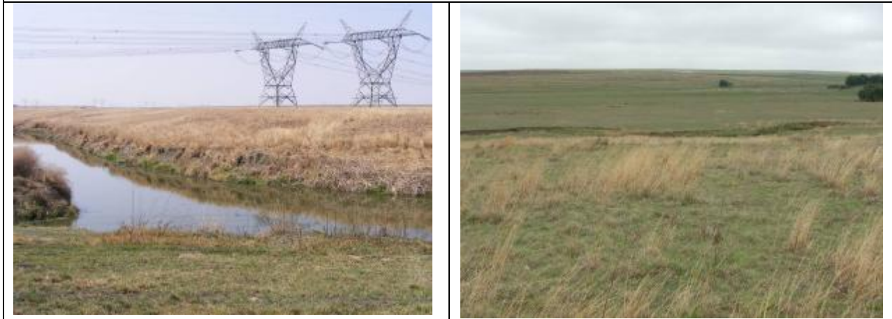
Waterval River showing existing power line crossings
