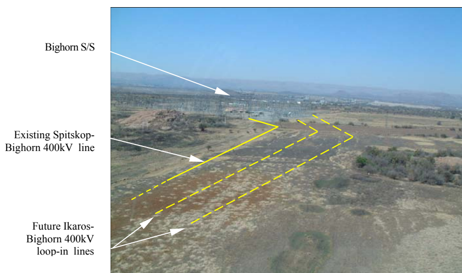
Figure 1.4: Aerial photograph illustrating the existing and proposed Bighorn Substation outgoing lines (Clara, 2001)
