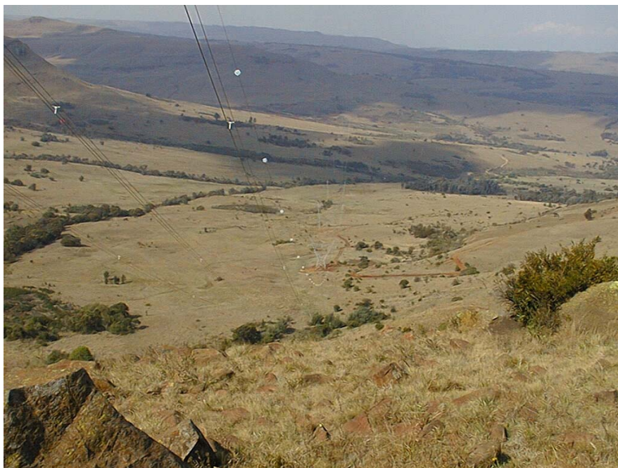
Figure 4.2: Bird diverters have been developed and have effectively reduced the incidents of bird collisions with Transmission lines
