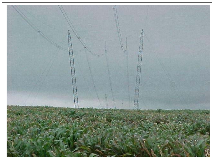
Figure 4.4: Use of the cross-rope suspension tower will enable landowners to use valuable agricultural land around the smaller footprint of this tower type
