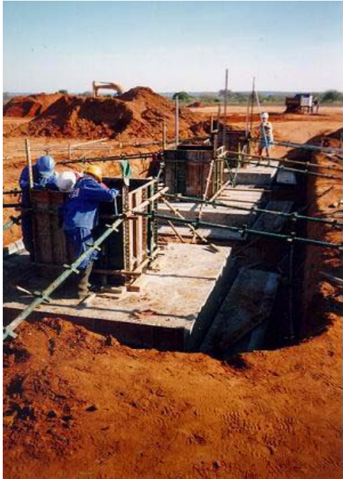
Photos 2 and 3: Example of transformer foundations
