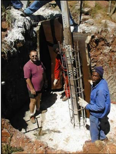
Photos 7 & 8 Pylon foundation (strain / bend type tower) and pylon foundation structures
