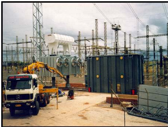
Photos 4 and 5: Example of transformer installation
