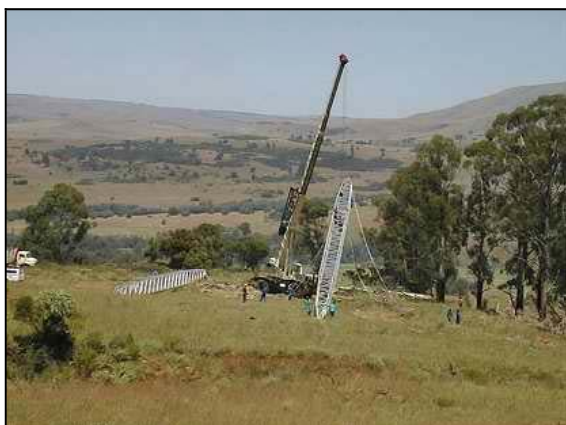
Photo 9 Lifting of structures for lattice – type transmission line towers
