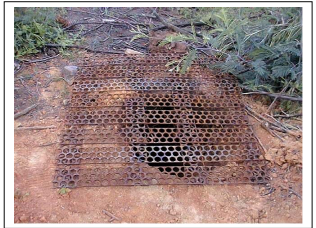
Photograph B4: Cover over foundations
