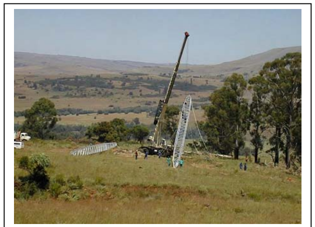
Photograph B6: Erection of towers by crane
