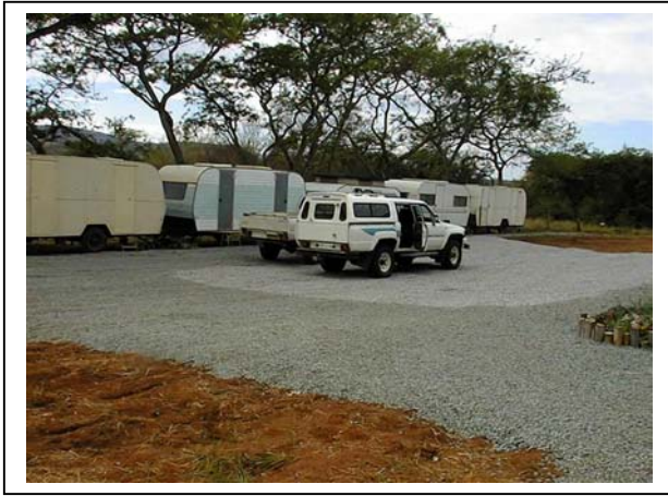
Photograph B1: Typical construction camp
