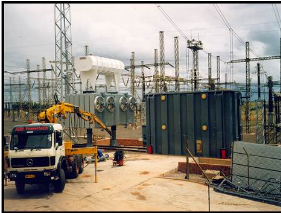
Photos 5 and 6: Example showing transformer installation
