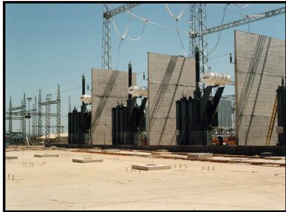
Photos 5 and 6: Example showing transformer installation
