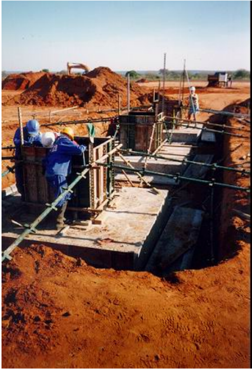
Photos 3 and 4: Examples of transformer foundations
