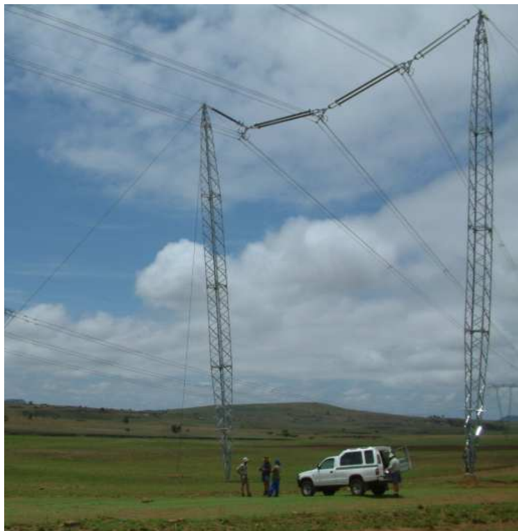
Figure 29: Cross-rop suspension tower
