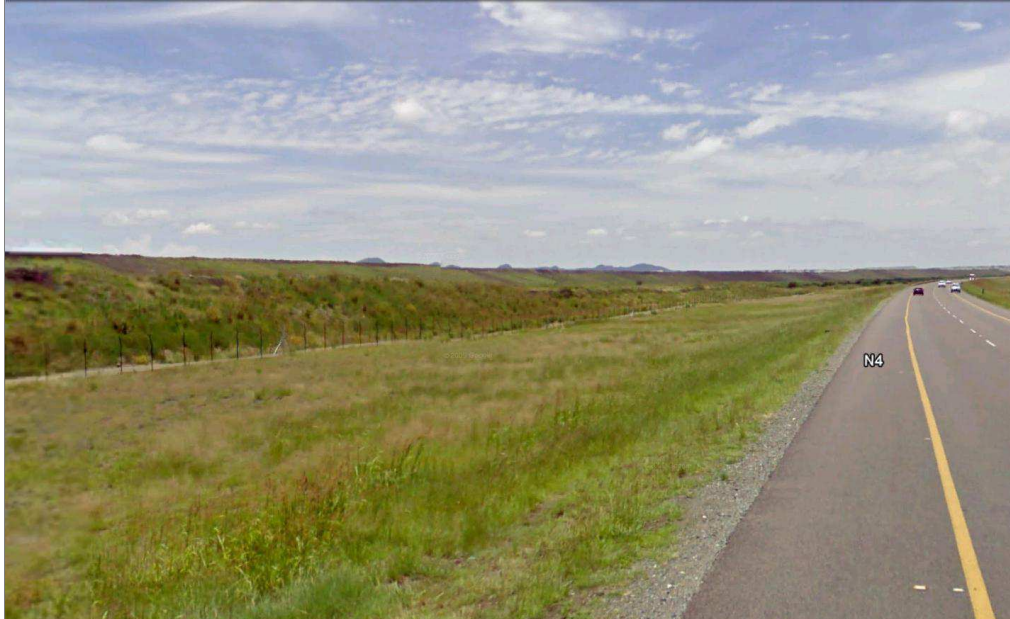
Figure 25: North-eastern view along the Western Route Alternative – Deviation 2 - route situated between the slimes dam (left) and the N4 (right)
