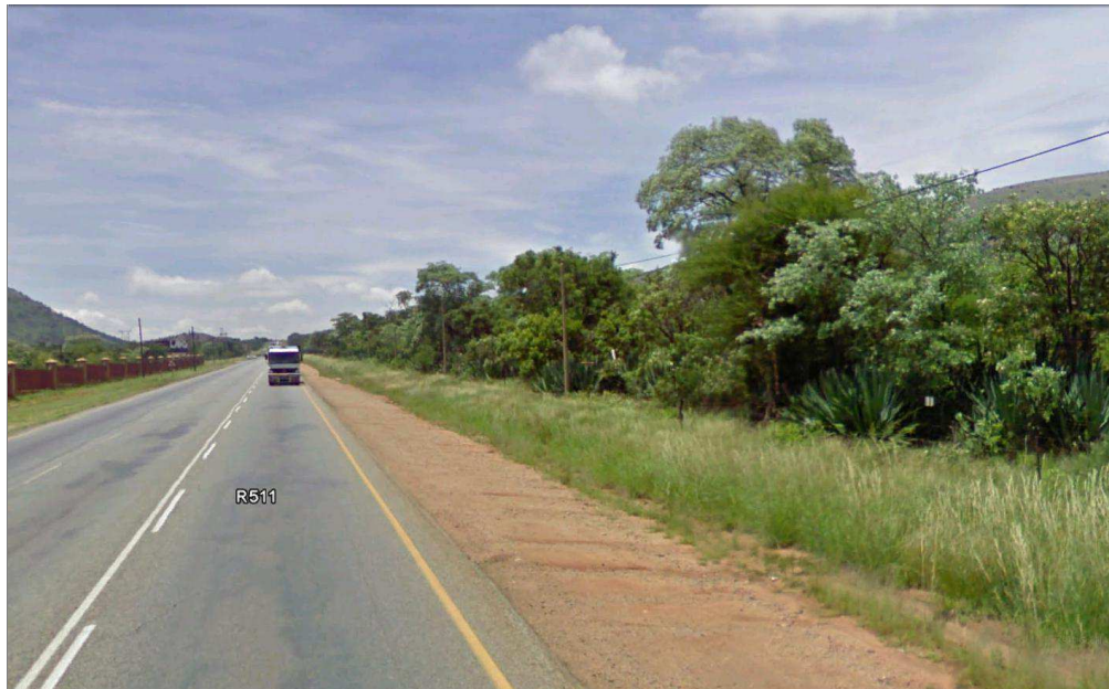
Figure 27: South-eastern view along the Western Route Alternative – Deviation 3 - route situated to the right of the R511
