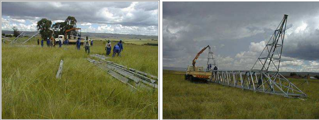
Figure 39: Delivery of steel (top) and assembly of tower (bottom)
