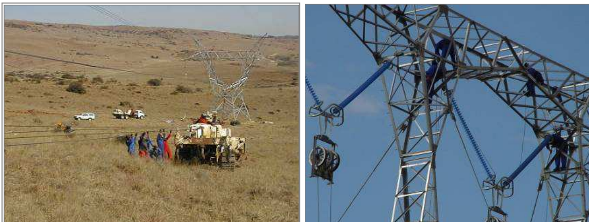
Figure 42: Stringing with pilot tractor (top) and pulleys (bottom)
