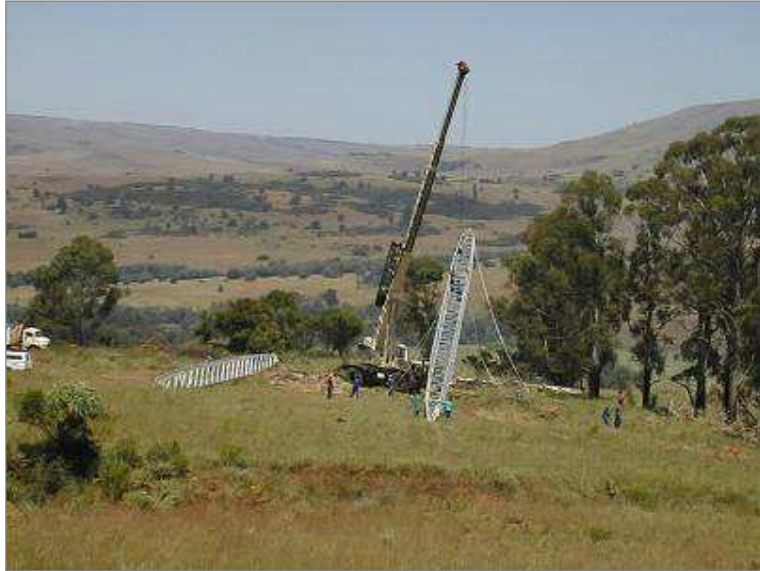
Figure 40: Erection of towers
