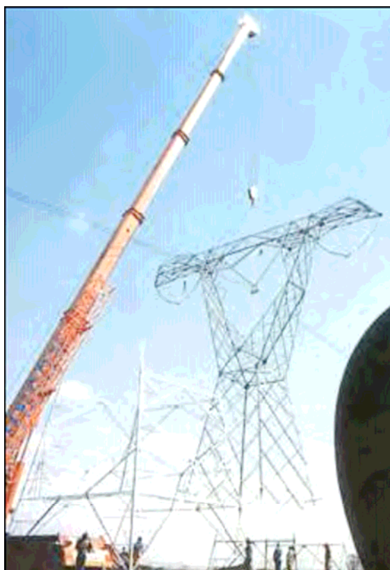
Figure 13 Illustration of a crane lifting the tower into place
