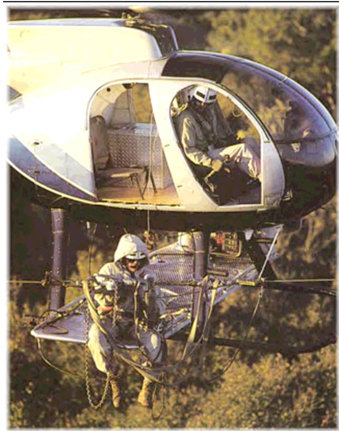
Figure 14 Maintenance undertaken by helicopter
