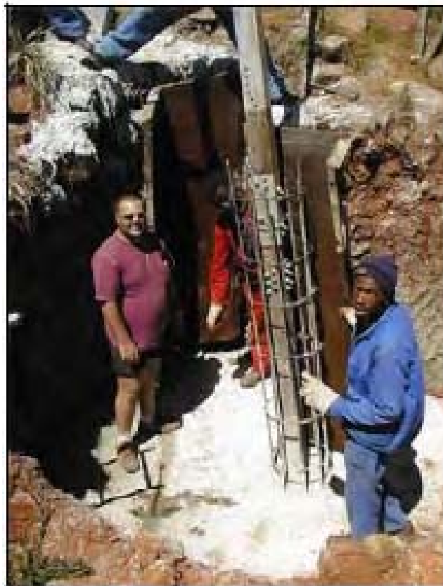
Figure 11 Pouring of concrete into the tower foundations
